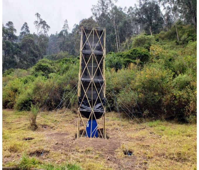
Fig. 7 Condensation tower design
