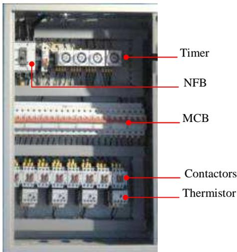
Fig. 8 Aeration control module
