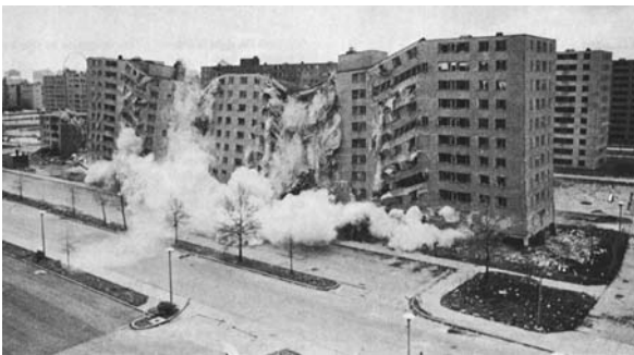
Fig. 3 The demolition of Pruitt-Igoe apartments
