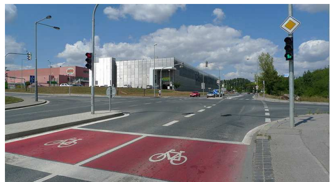
Fig. 2 Bike boxes without the approaching lane [19]
