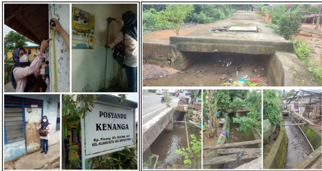
Fig. 2 Flood Inundation Height Location, Documentation 2021
