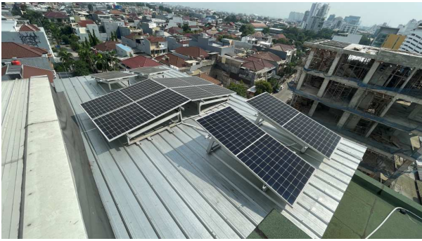
Fig. 5 Experiment of various solar PV orientation
