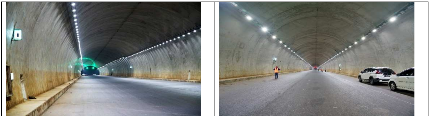
Fig. 2 Inside Cisumdawu Tunnel
