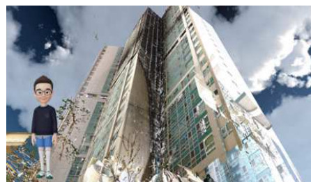
Fig. 3 Scanning the Exterior of the Fire Scene
