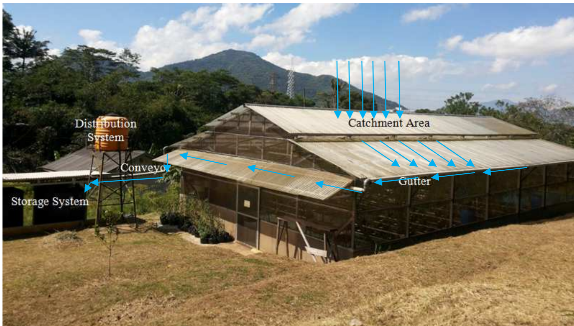
Fig 1. Rooftop Rainwater Harvesting System for Agriculture
