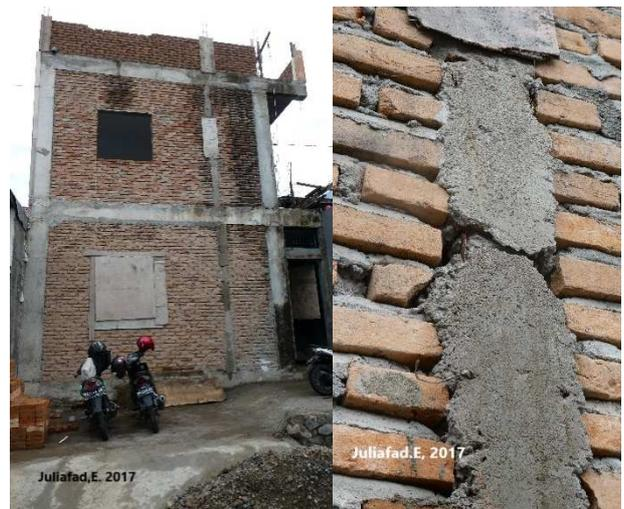
Fig. 13 Sample of structural defect due to improper compaction
