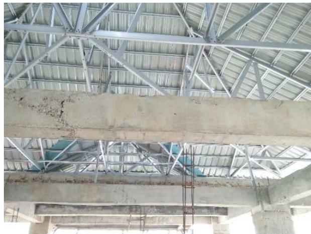
Fig. 17 Finding on concrete defect due to improper construction joint treatment
