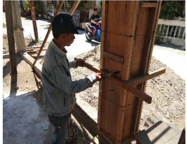
Fig. 12 One of the builders used hummer to compact the placed concrete
