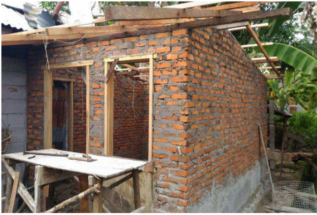
a. Brick Construction
