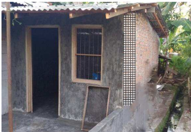
c. Mortar Construction
